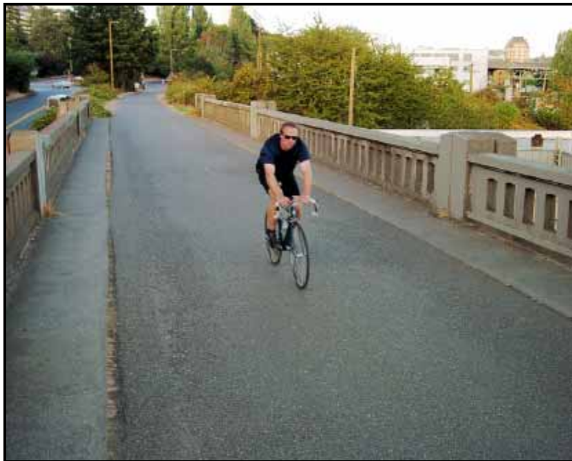
Figure 4.31 – Bridge with Additional Horizontal Clearance (Seattle, WA)
