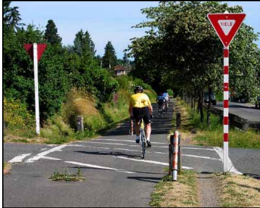
Figure 4.11 – Yield Signs at a Marked Pathway Crossing (Seattle, WA)
