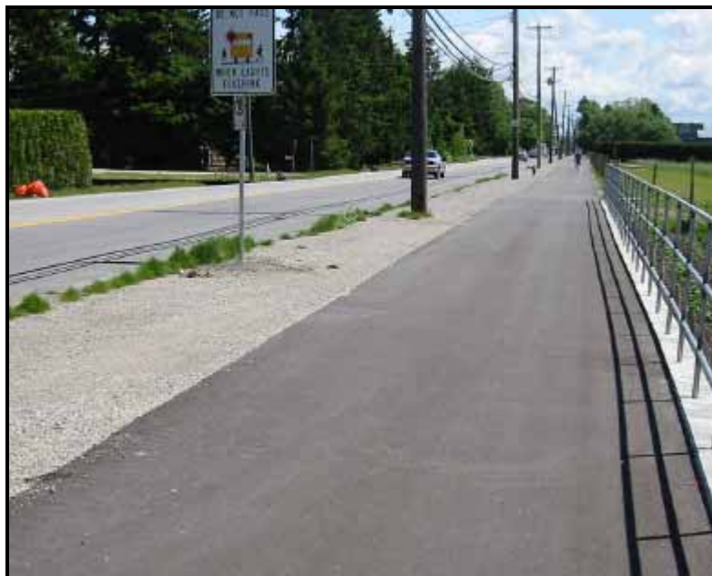
Figure 4.1 – Pathway Within Road Right-of-Way (Richmond BC)
