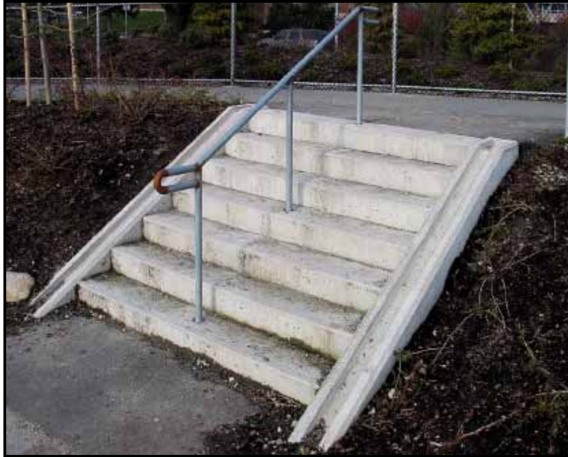
Figure 4.34 – Stair with Bicycle Ramp (New Westminster, BC)
