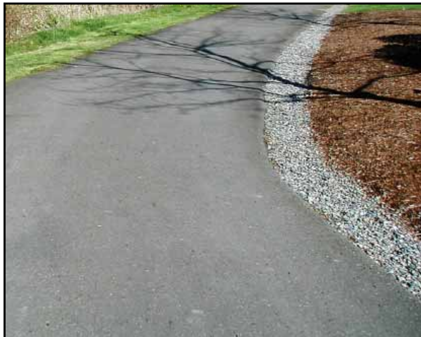
Figure 4.5 – Aggregate Pathway Shoulder (Tukwila, WA)
