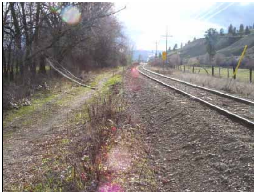
Figure 3.1 – Existing Rail Line (east of Dilworth Drive)
