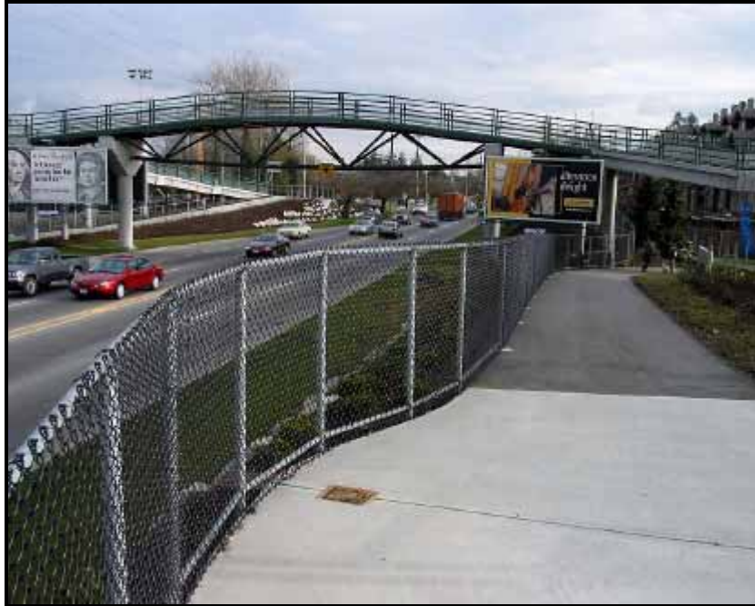
Figure 4.21 – Overpass (New Westminster, BC)
