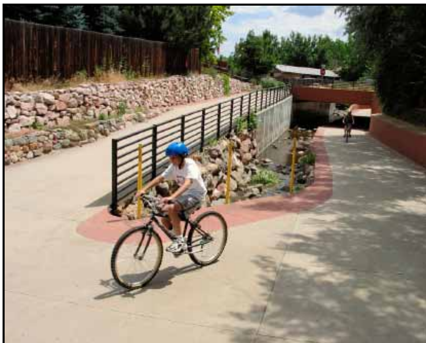
Figure 4.22 – Underpass (Boulder, CO)
