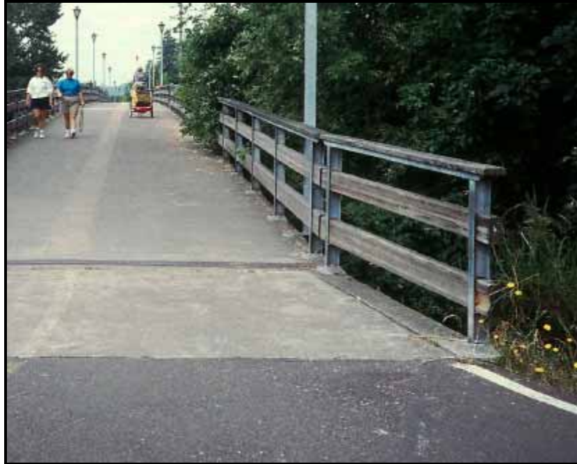
Figure 4.33 – Railing Flared at Bridge End (Eugene, OR)
