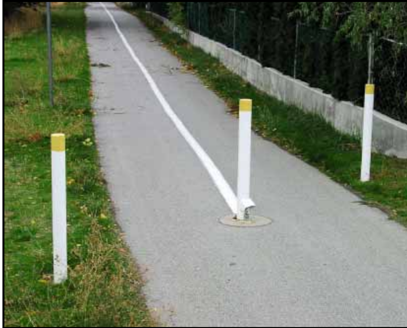
Figure 4.29 – Barrier Posts (Penticton, BC)
