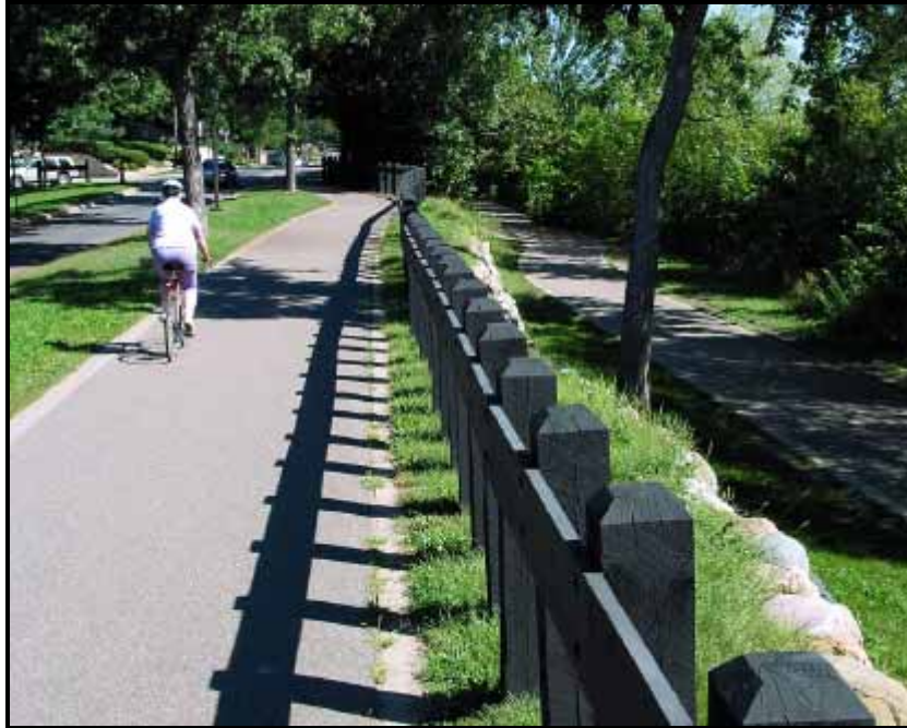
Figure 4.26 – Safety Railing Adjacent Steep Side Slope (Minneapolis, MN)
