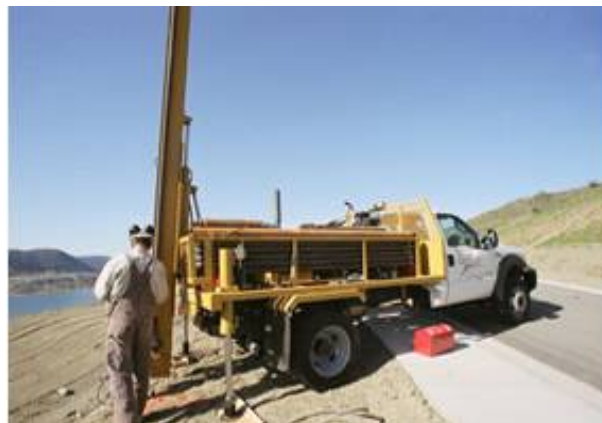
Geoexchange system under construction.
