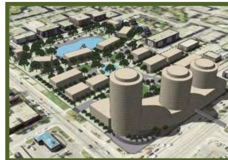
View from Northeast
