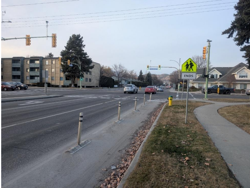
Figure 1. Example of flexible delineator posts
