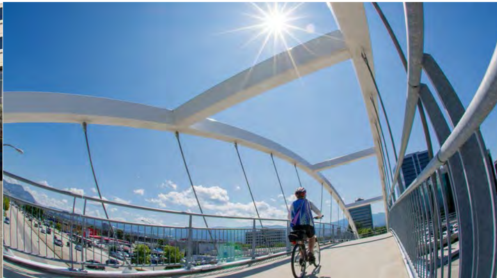
Pedestrian bridge to Landmark
