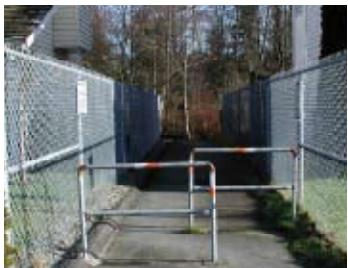
Generally, use metal bollards in more urban environments, and wood bollards in more natural settings or where a wood fence or railing is used at a trail head.
