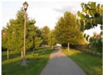
**Surfacing:** Ensure uniform consistent surface (well compacted for aggregate trails) without puddles or depressions and free of obstructions.
