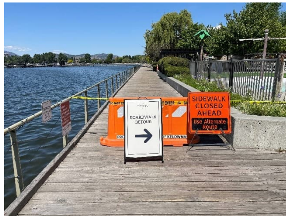
Figure 2-2 Boardwalk barricades in place
