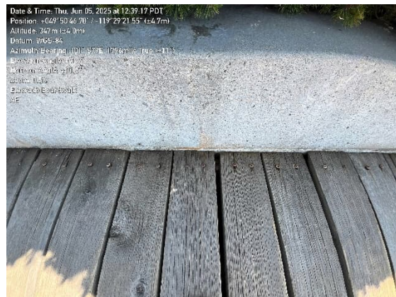
Figure 4-2 Deteriorated planks
