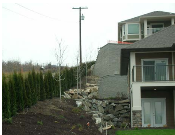
Retaining wall in appropriately used to improve views and create a flat rear yard
