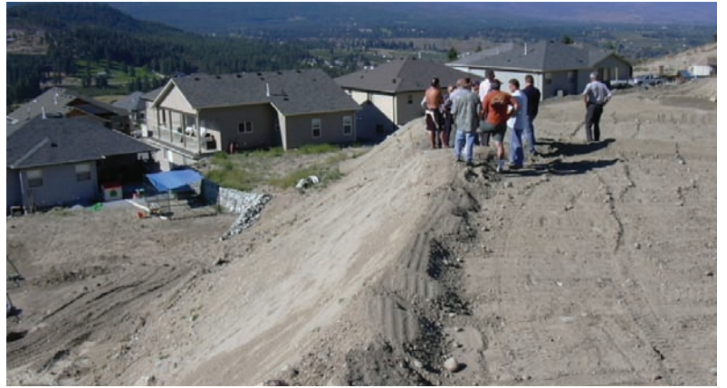
Potential slope instability
