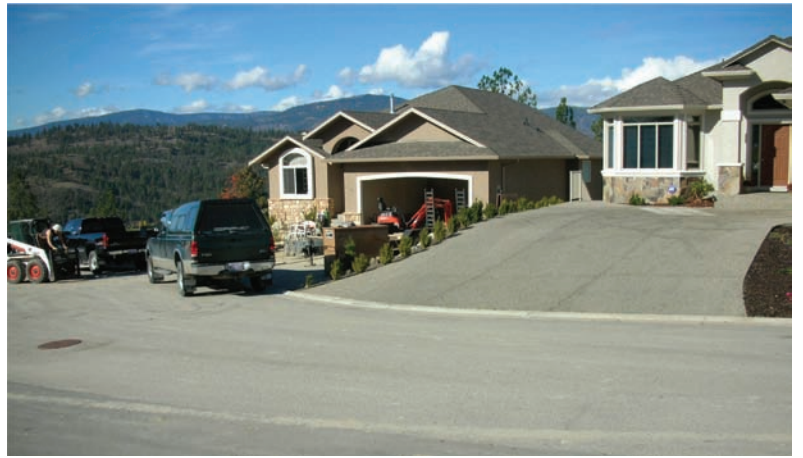
Driveway slope does not respect natural terrain
