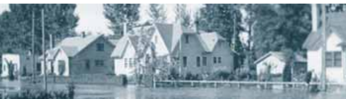
Spring flooding on Marshall Street c. 1940s. Flooding was an annual event as Mill Creek overflowed its banks each spring, and groceries were sometimes delivered in a canoe. In the 1990s the city installed a diversion system which reduced the flood risk for residents.
