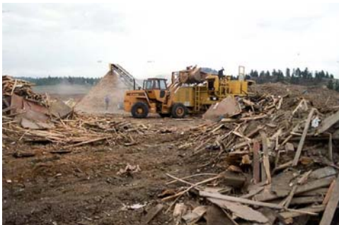
Wood Chipping at Landfill
