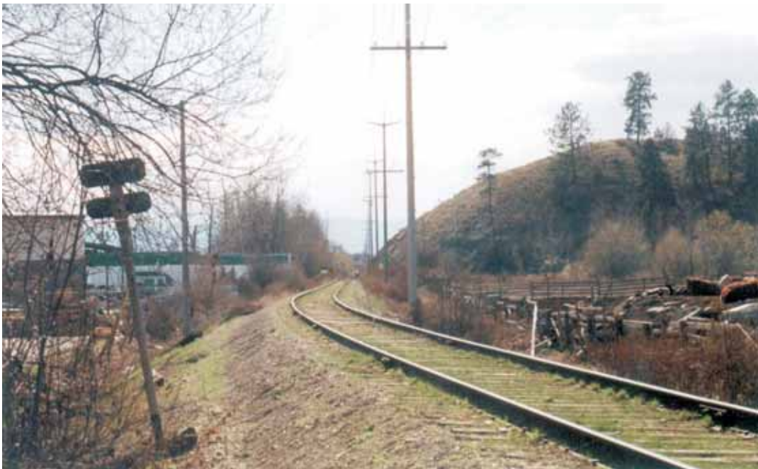
FIGURE 1.3 NEAR McCURDY ROAD, FACING SOUTHWEST
