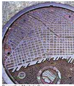
Decorative Manhole Covers
